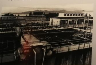
供水厂 Water Supply Plant
